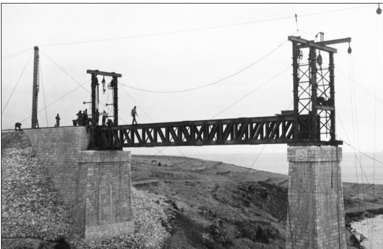
Nahr El Djadz - Image 4: The nose has gone, the cribs have been removed and the first (south) span has been lowered into its final position. Photo: ARHSnsw.
