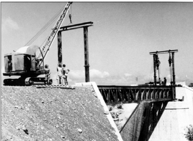
Nahr El Fgal - Image 5: A mobile crane places steel rail as ballast to balance the span until the nose reaches the other abutment. Photo: ARHSnsw
