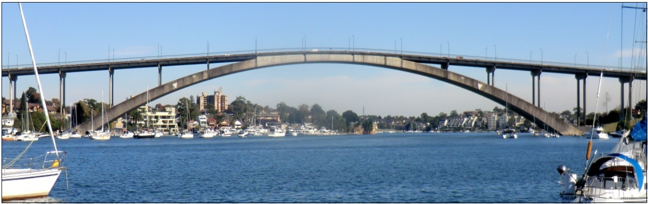
The Gladesville Bridge, viewed from the north-east.
