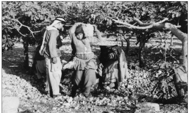
Track ballast was obtained by our machines, and local piece-work. Here, gang of Bedouin women also assist in gathering and carrying stone from adjacent olive groves, while an Arab Rias (ganger) supervises.
