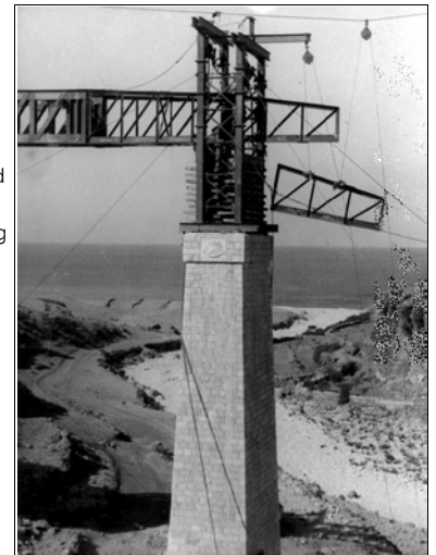
Nahr El Djadz - Image 1: The first span on wheeled trucks is ready for pulling forward. Note the light weight launching nose and the ballast, of spare rail, at the rear to ensure that the nose reaches the next pier before the whole lot tips over. Photo: ARHSnsw
