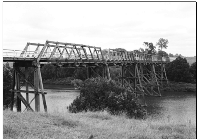
The Killawarra Bridge over the Manning River near Wingham NSW. One of my sad failures, demolished circa 1986. Photo: MJ Doring, 1985.
