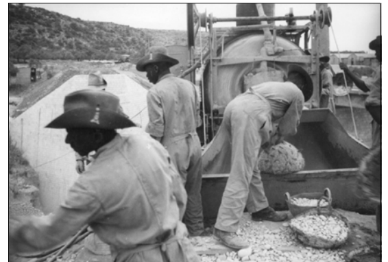
South Africans loading the concrete mixer with coarse aggregate supplied in baskets. This is probably the Nahr El Fgal bridge. Photo: ARHSnsw.
