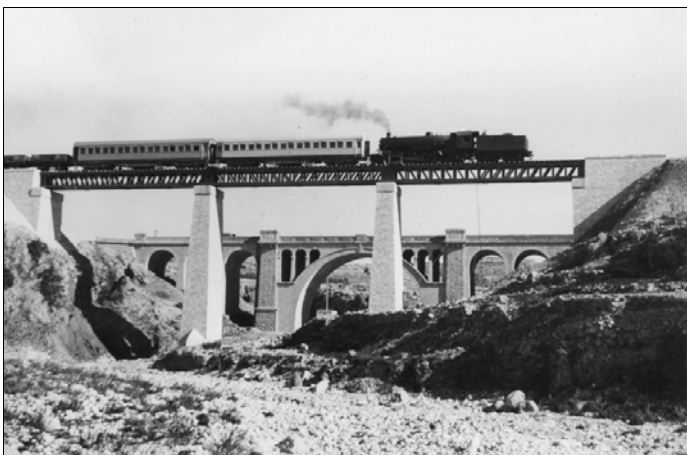
Nahr El Djadz - Image 4: The nose has gone, the cribs have been removed and the first (south) span has been lowered into its final position. Photo: ARHSnsw.
