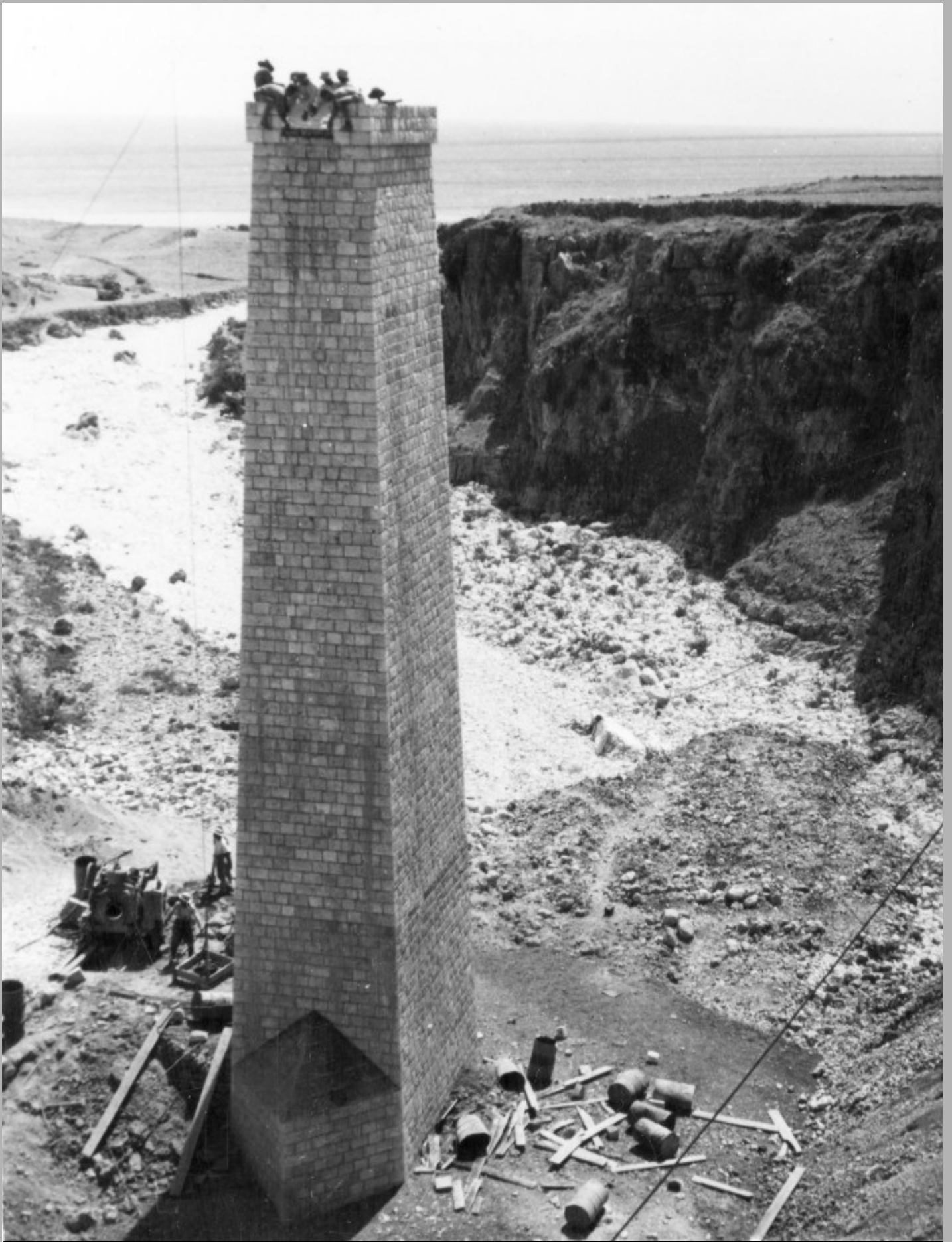
On the Beirut to Tripoli Railway – the first 98 foot (about 30m) high pier of the Nahr el Djadz (No.1) bridge has been completed. A group of men on the top are installing the "piece de resistance" of the pier – a carved stone AIF rising sun badge – to be seen by passers by from the road bridge to the east, where the photographer is probably standing. To the west is the dry river bed and the Mediterranean Sea beyond.
