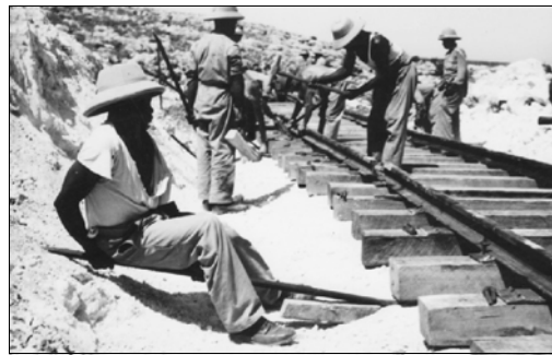
South Africans laying tracks north of Maameltein. Photo: ARHSnsw.
