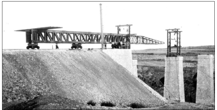
Nahr El Djadz - Image 1: The first span on wheeled trucks is ready for pulling forward. Note the light weight launching nose and the ballast, of spare rail, at the rear to ensure that the nose reaches the next pier before the whole lot tips over. Photo: ARHSnsw
