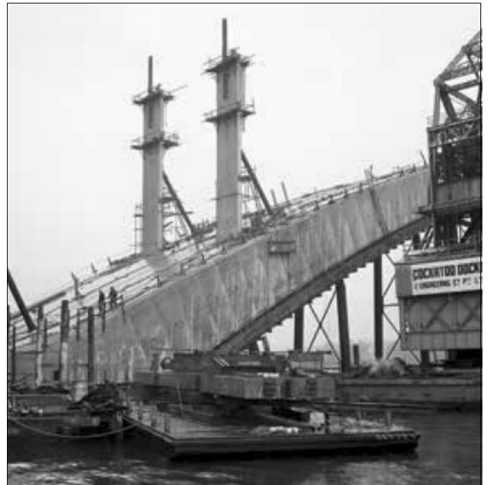
A pair of columns is in place on the arch, ready for installing a pre-cast headstock. Photo: RTA - no date or number.
