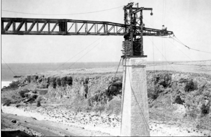
Nahr El Djadz - Image 2: The limitation of launching a single span was that the launching nose then extended out of reach. It had to be dismantled for the next use, piece by piece, high in the air using a block and tackle extending from the lowering gantry. Photo: ARHSnsw.
