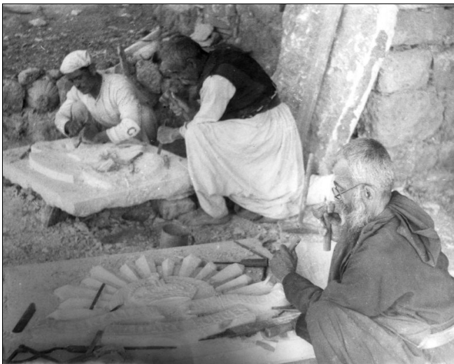
Carving Australian Rising Sun Plaques for bridge piers. At right is Brother Natamuk an altar sculptor from the Maronite church at Byblos and two assistants. Bro. Natamuk selected the stone from the nearby mountains, and our railway draughtsmen made templates for the sculptors' guidance. The accuracy and gleaming finish of the plaques is a tribute to these Lebanese craftsmen. The largest plaques were approx. 4 ft. x 3 ft.
