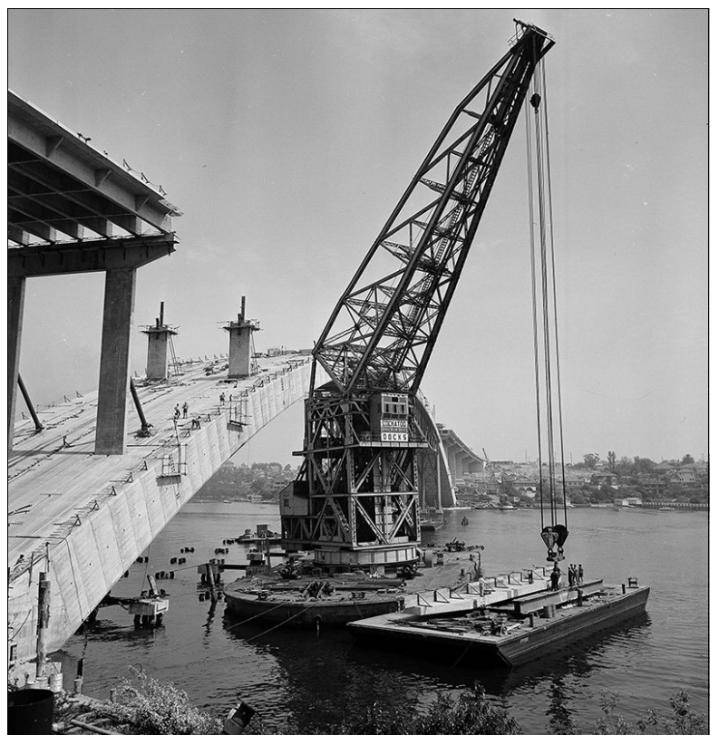
A pair of columns is in place on the arch, ready for installing a pre-cast headstock. Photo: RTA - no date or number.
