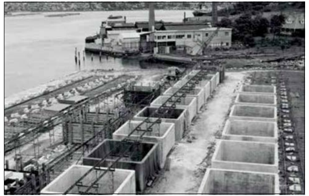
Box units in the casting yard at Woolwich. Photo: RMS January 1962.
