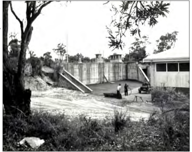
A 1965 view of the only visible external wall of the bunker. A storage shed on the right dates from 1965. Source: WA Dept of F&ES.
