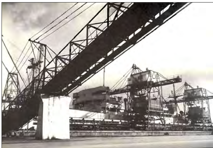
Coal Unloaders and Conveyers, Metropolitan Gas Works, West Melbourne, 1933. Designed by Albert Longoni, built by Malcolm Moore Ltd.
