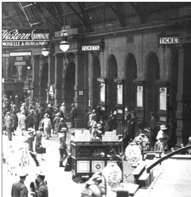
This detail from the 1927 Sam Hood cover image shows the 4 large cabinets and 4 small ones underneath them, all fixed to the north wall of the Concourse. The pedimented doorway to left of the boards, leads to the Central Tram Station overlooking Eddy Avenue.
