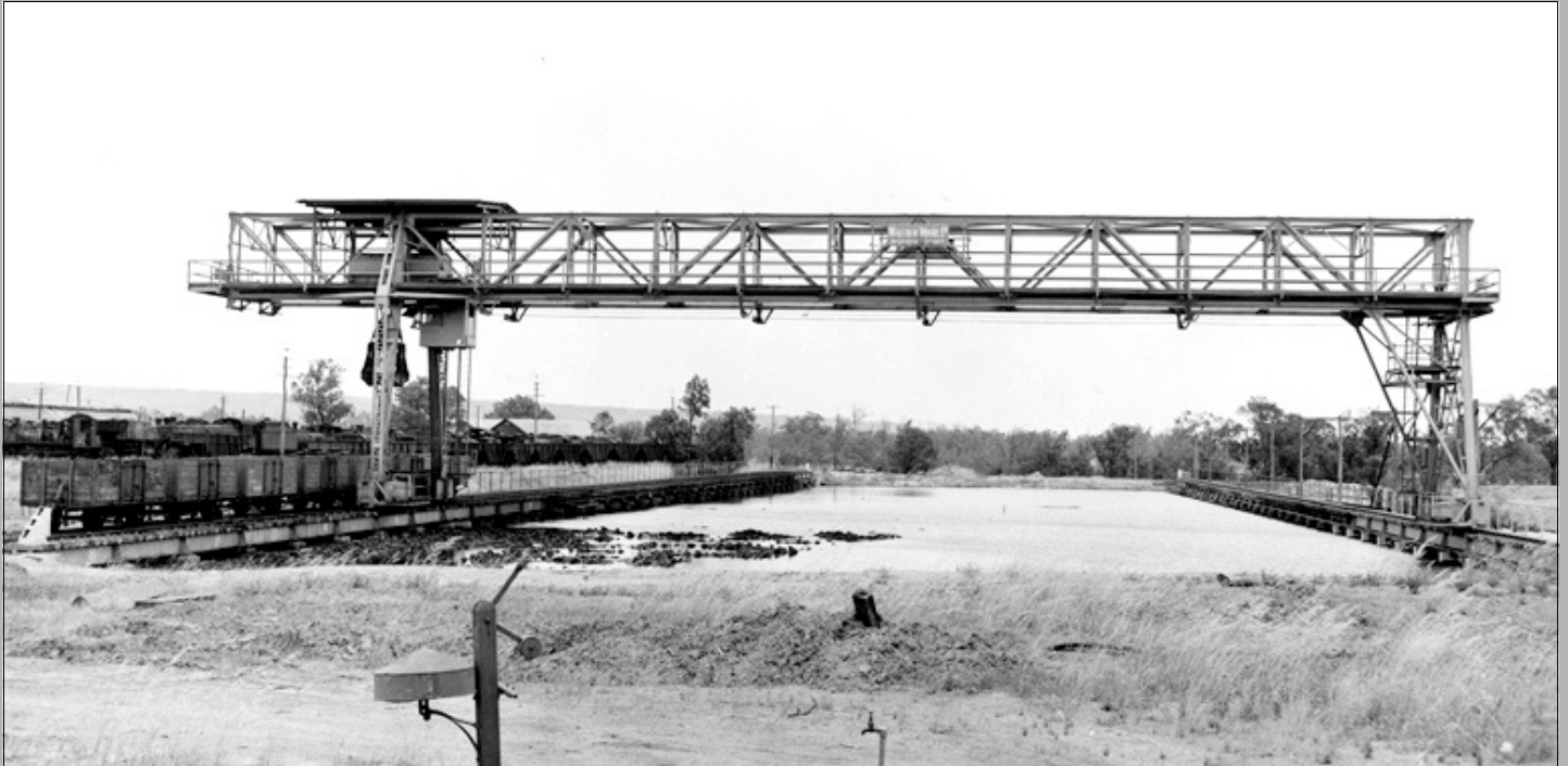
Image Above: Malcolm Moore Ltd Gantry Crane on the Coal Dam at Midland Railway Workshops in WA.
