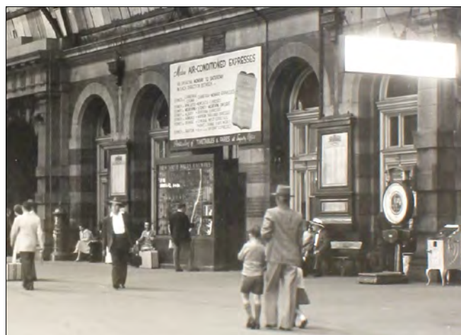
Only two of the Honour Boards survive in situ in 1958. Source: NSW State Archives.
