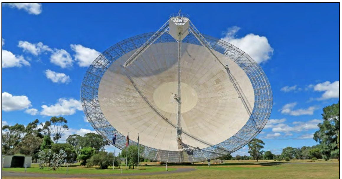
Image at Right: The modern Parkes Telescope photographed on 3 March, 2022. The dish surface as it appears today, after the last of the surface upgrades and with the new 3-sided focus cabin. Photo: John Sarkissian.
