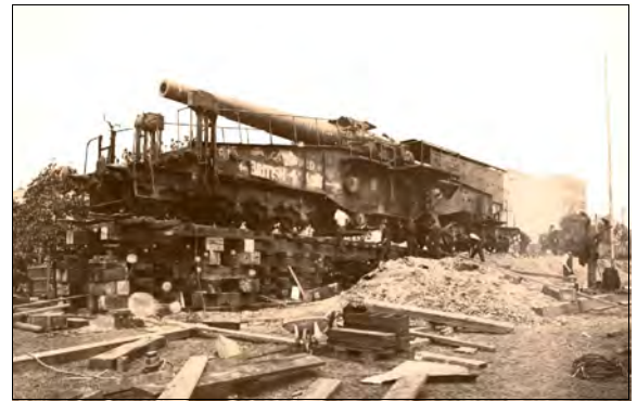
Rerailing the gun with jacks and pigsties. April 1920.
