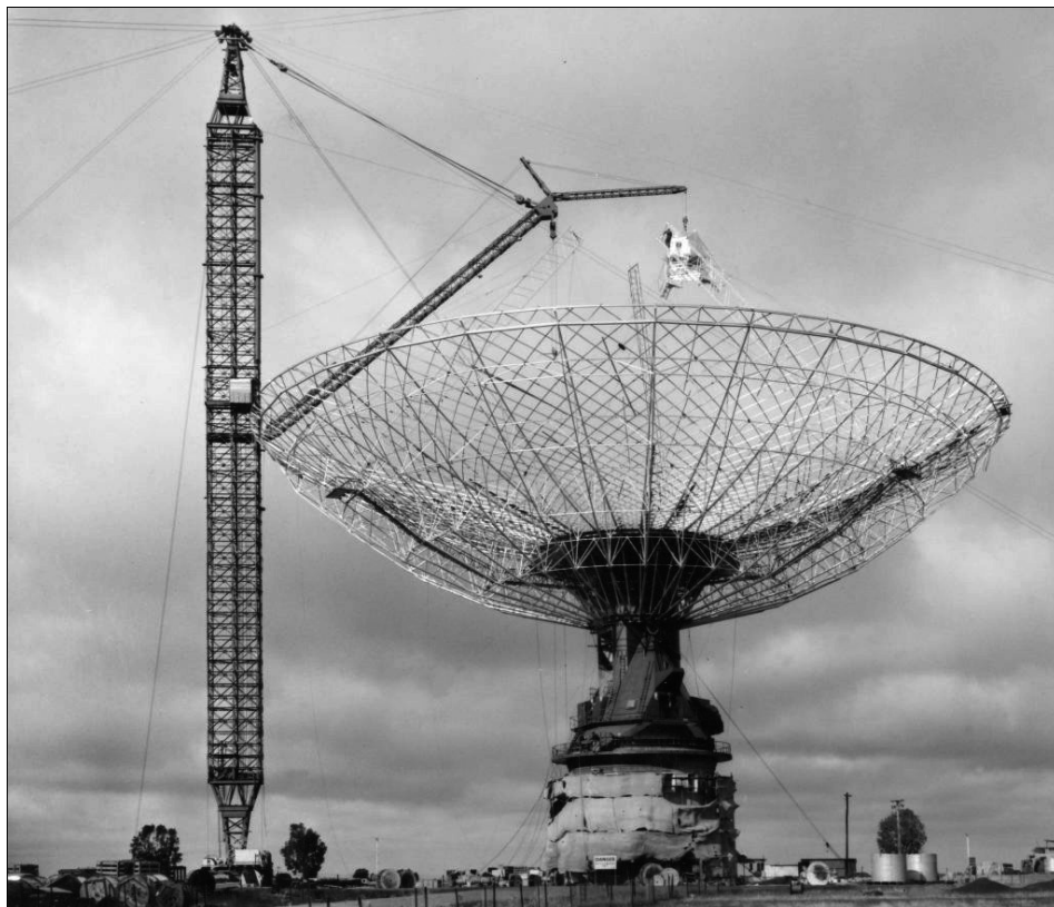
Parkes Radio Telescope under construction circa 1961.
