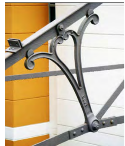
A replicated lily-flower strut as used in the re-erected Grissell Building. Photo: ICS.
