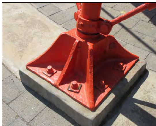
Iron Lighthouse Port Adelaide, base detail of the 1875 frame. Photo: Miles Lewis.
