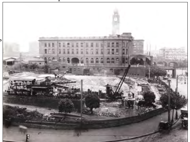
The gun is moved forward to clear construction work on the City Railway on 16 th November 1922. Soon embankments and retaining walls will rise, precluding removal of the gun.
