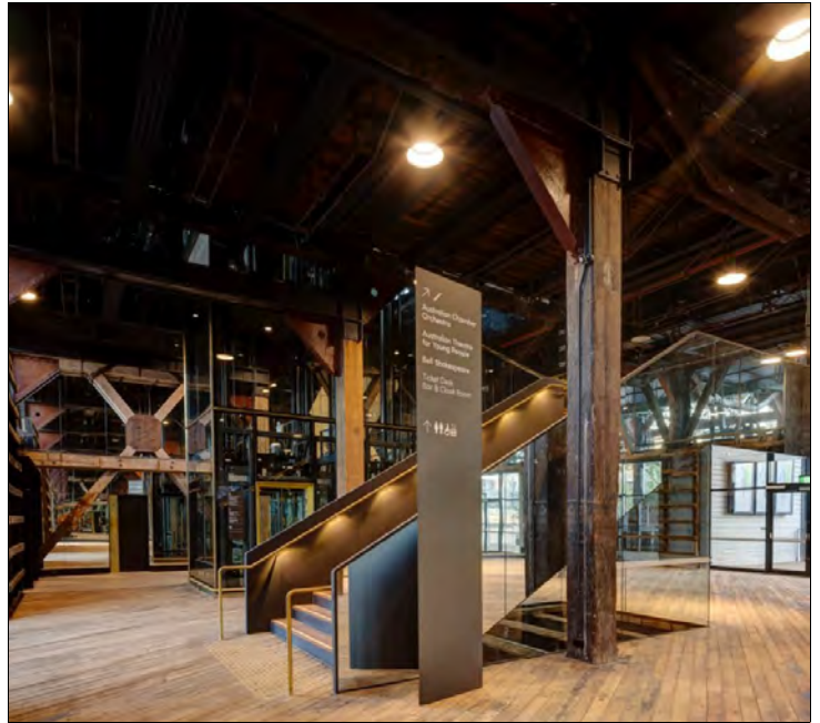
The shared Foyer at wharf level in Pier 2/3 with new lifts and stairs carefully inserted, and the conserved steel strongbacks. Photo: Brett Boardman.
