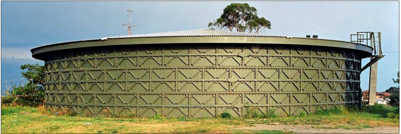
Cast iron reservoir made for the Walka Water Works by the Birtley Iron Co, Newcastle, UK, c 1877, now at 147 Ocean St, Dudley, near Newcastle, NSW. The reservoir was still in use and well maintained when it was photographed in 1992. Photo: Margret Doring, 1992.
