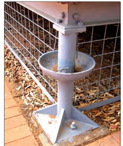
London & Hamburg Gold Recovery Co.. assay office, vermin-proof pillar: Photo: Miles Lewis.
