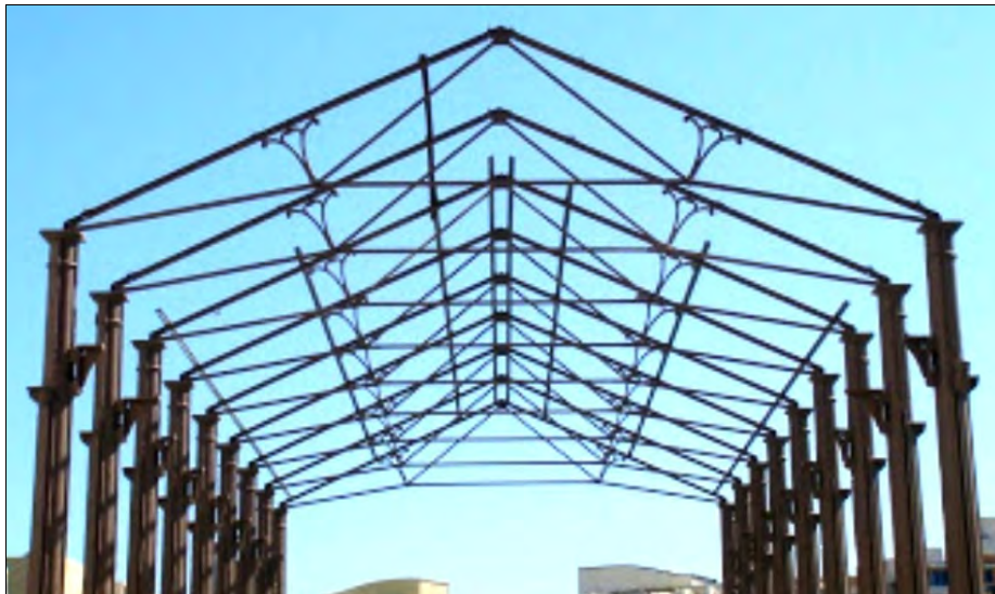
The re-erected nave of the Grissell building.
