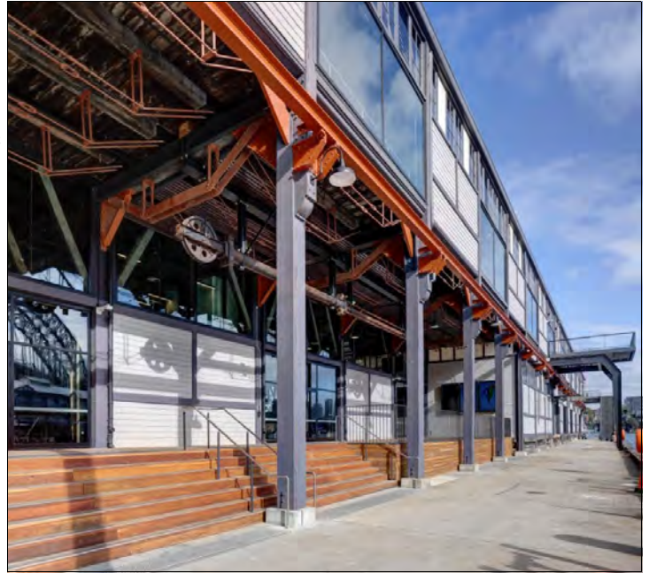
The conserved wharf exterior showing the gantry rail and a reconstructed gantry balcony. Photo: Brett Boardman.
