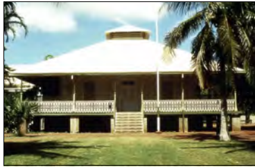
The Broome Cable Repeater Station (now Courthouse). Photo: Brian Kidd.
