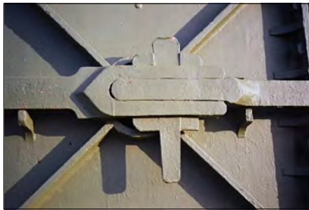
Joint in a malleable iron strap, Dudley Reservoir. Photo: Margret Doring, 1992.
